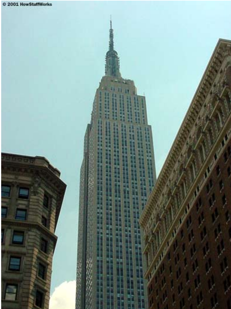
Figure 5: The Empire State Building's 73 elevators can move 600 to 1,400 feet (183 to 427 meters) per minute. At the maximum speed, you can travel from the lobby to the 80th floor in 45 seconds. Photo and caption copyright 2001 by HowStuffWorks, fair use for educational purposes.
